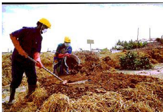
Fig. 1 - Compost and admixtures being laid layer by layer
