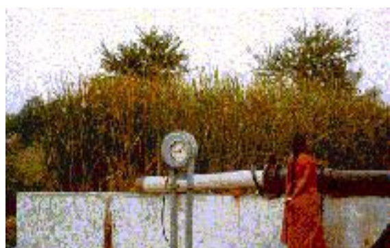
Picture 6: Reed bed developed at CETP-SIDCO
