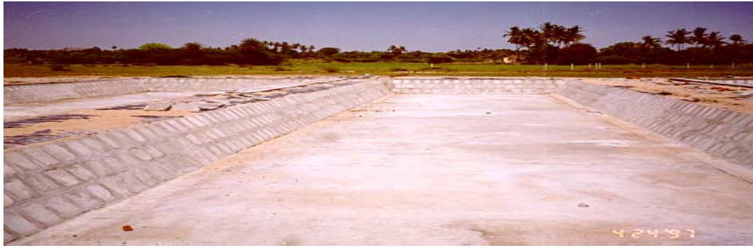
After concreting bottom & sides
