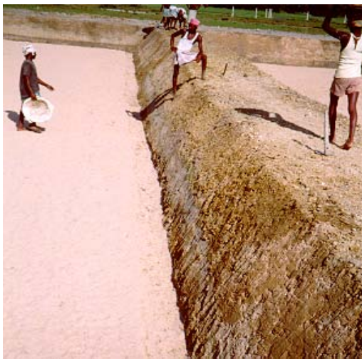
Filling first layer of sand
