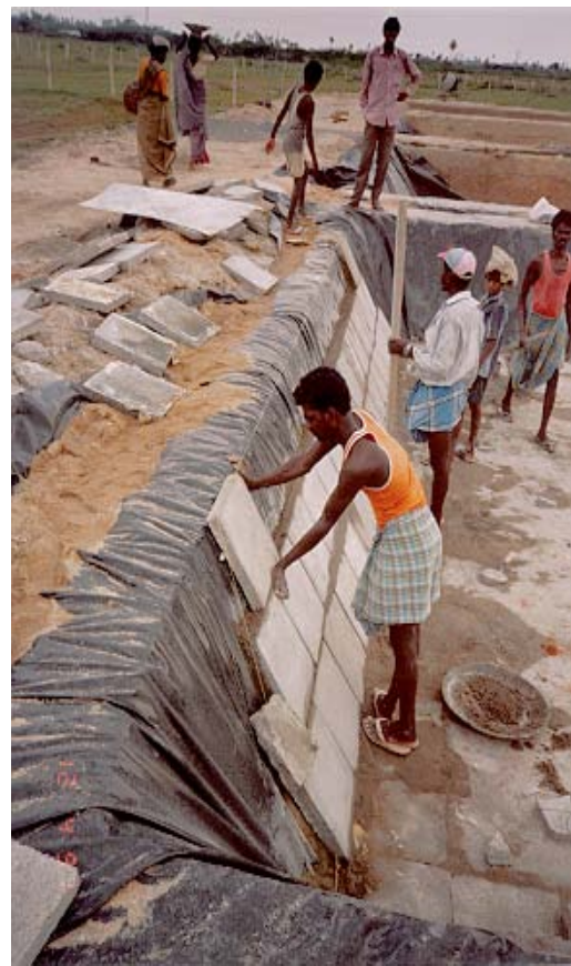
Fixing concrete slab on sides
